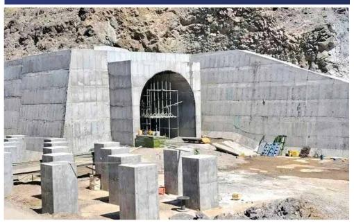
Significant progress has been made on the Bakhshabad Dam Farah province, project in western Afghanistan. According local officials. to 100-meter-long diversion tunnel has been completed, adhering to construction standards. all Additionally, the concreting of one
